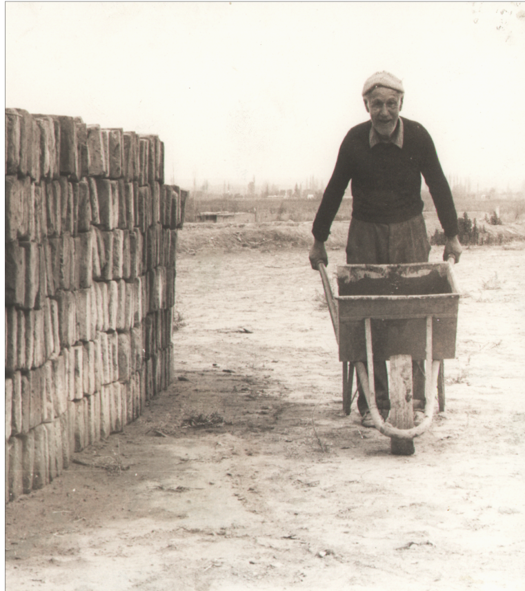
Student project 1987: We have built up the frame of the community house and casted the floor. Don Juan – one of Branden's oldest residents – was always there with us working. One of the inhabitants proved to be good at plastering and led the work on making a nice colored cement floor surface. Photo: Stenberg & Kain, the photo of Don Juan probably Sergio Aguirre.
