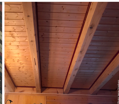
Re-used ceiling beams.
